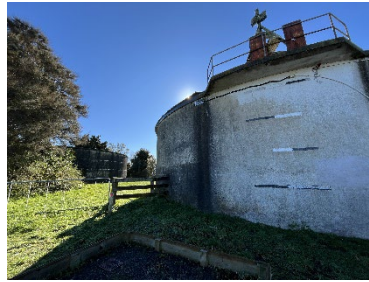
Thomson Ave Reservoir
