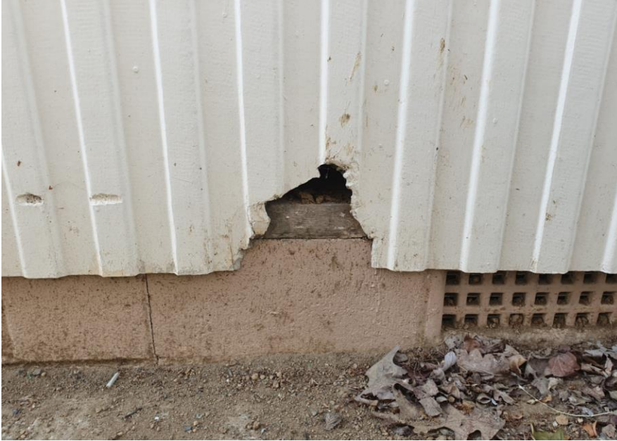
Figure 3: Example of damaged ACM cladding
