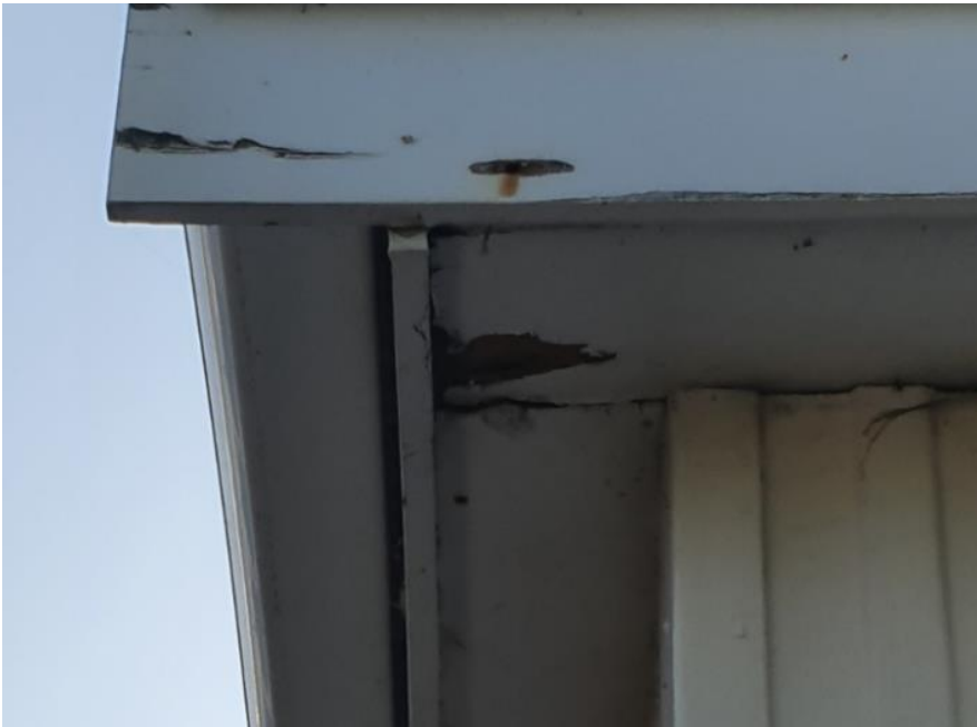
Figure 2: Example of rotting exterior timbers
