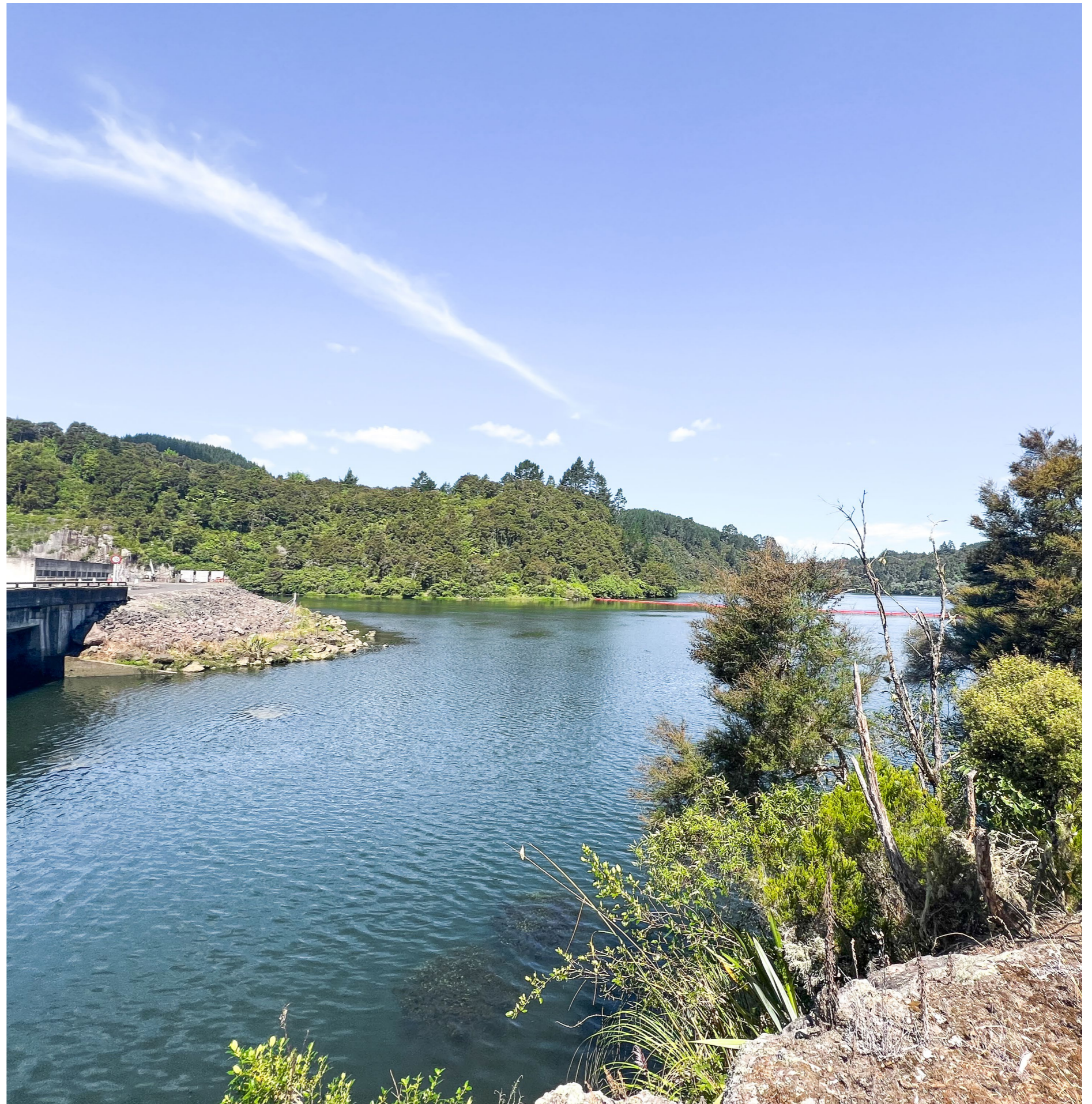
Figure 18. View of Waipapa Dam
