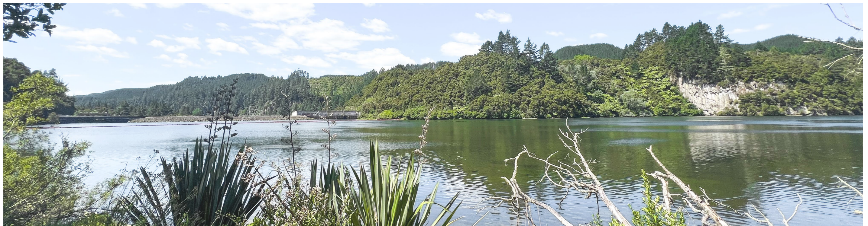
Figure 1. View of Waipapa Dam
