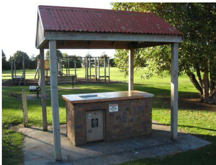
Example - Single hotplate bricked in unit – Leamington Domain (bench is part of brickwork)
